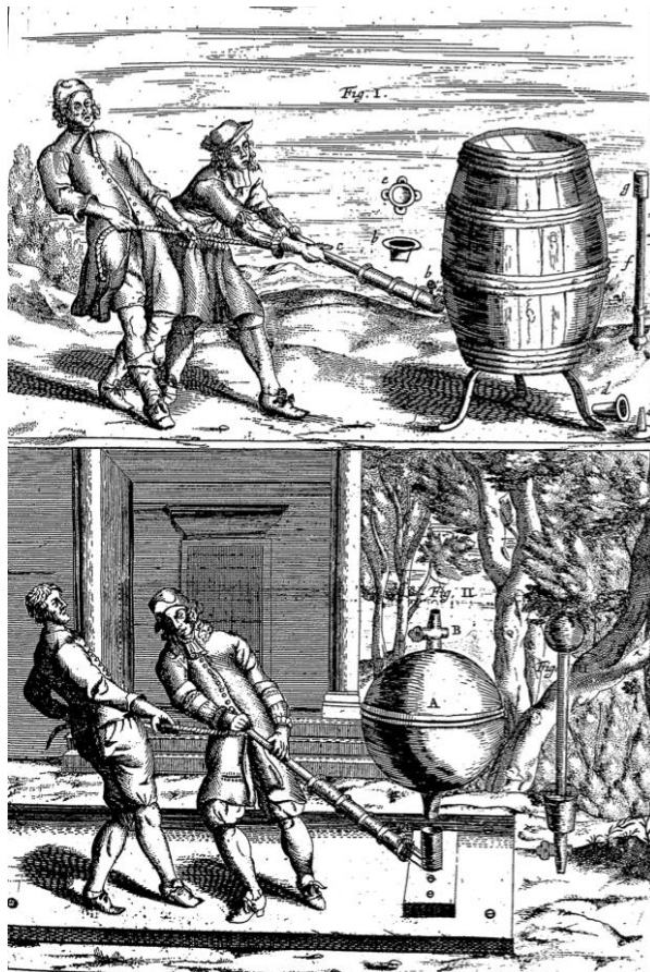
Figure 1. Experiments with a wooden barrel and metallic hemispheres. (Guericke 1672, 74)
